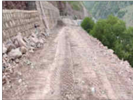
Construction of a permanent access road at the dam site
