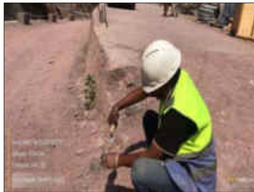
Soil sampling at the A2 camp ( June 2024)
