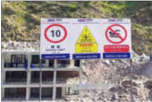
Signage installed at the dam site
