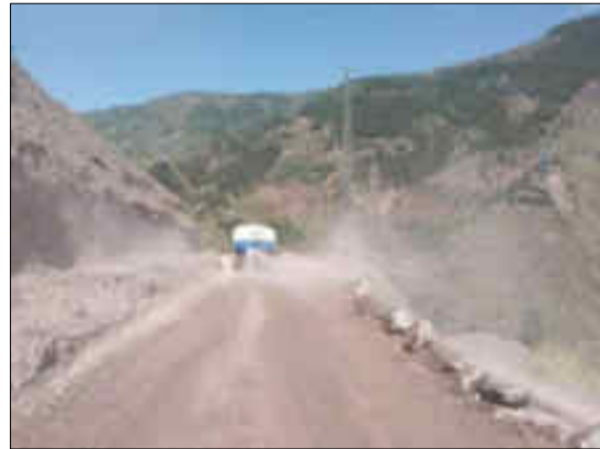
Water sprinkling at the A3 access road
