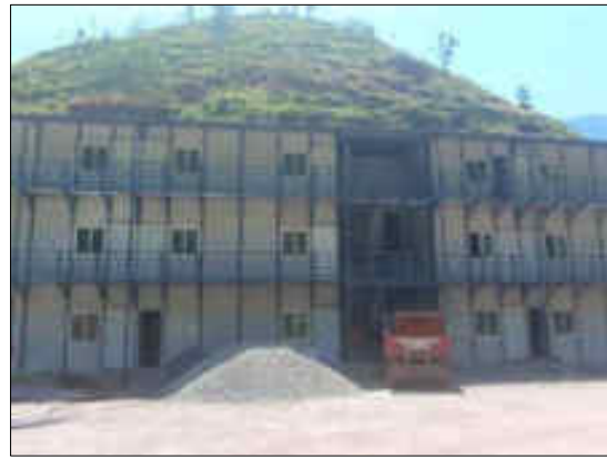
EPC Contractor's camp construction at the A3 site
