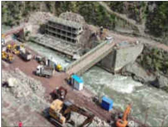
Overview of the dam site construction activities
