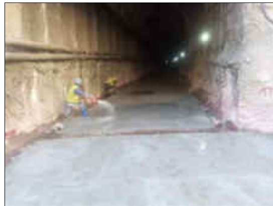
Adit 2 invert concreting
