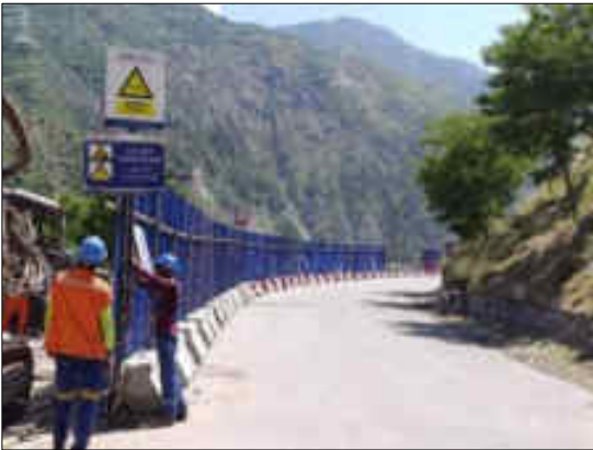
Construction site barricading at N-15 (dam site)
