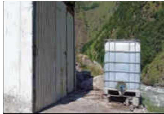
Provision of a latrine facility at the dam site
