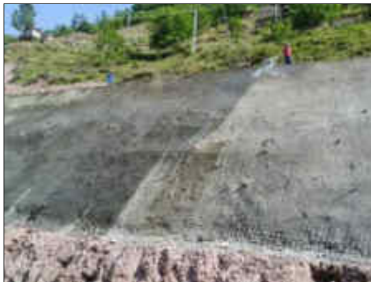
Shotcreting at slopes for stability at the dam site
