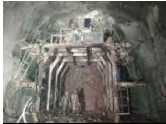
Excavation and support work at Adit 3
