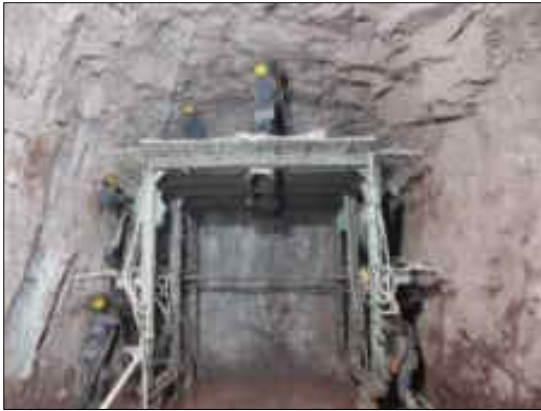
Excavation and support work at Adit 1
