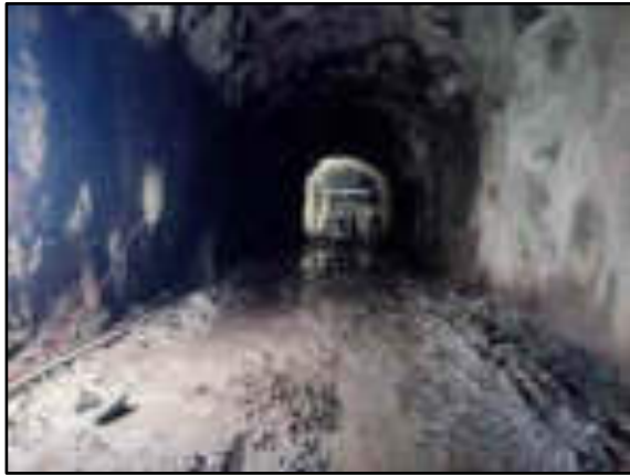
Construction Works at Adit Tunnel-01
