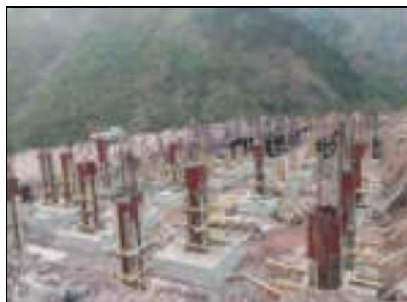
Construction Works at Residential Colony
