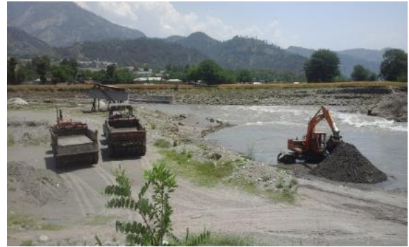
Sand mining with excavator
