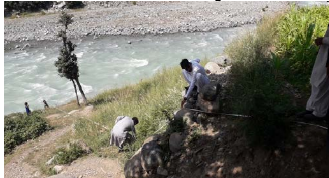
DMS at Powerhouse site
