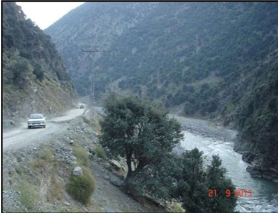
Figure 2.8: Proposed Weir Site Location PS Hydropower Project near Patrak Village (towards upstream of weir location)
