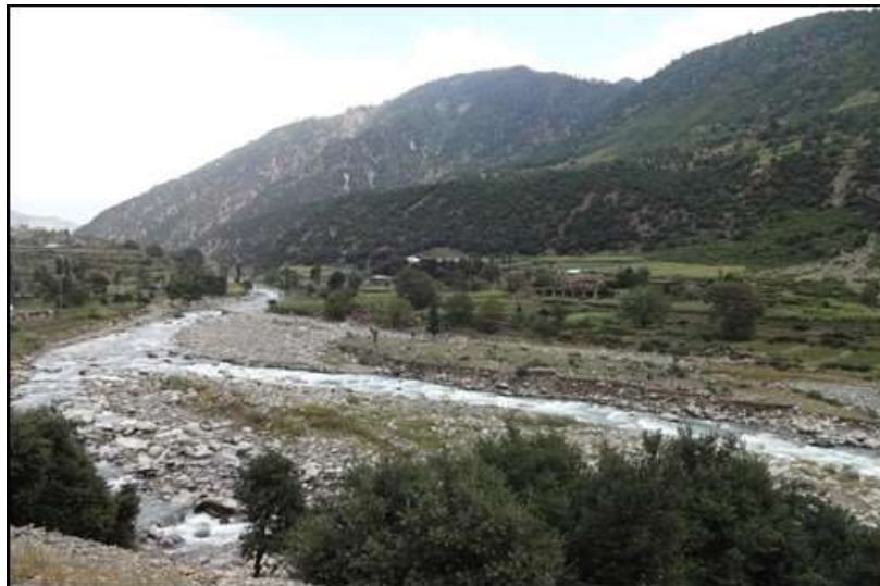
Figure 2.6: Proposed Weir Site Location KBP Hydropower Project near Kalkot Village (towards upstream of the weir location)
