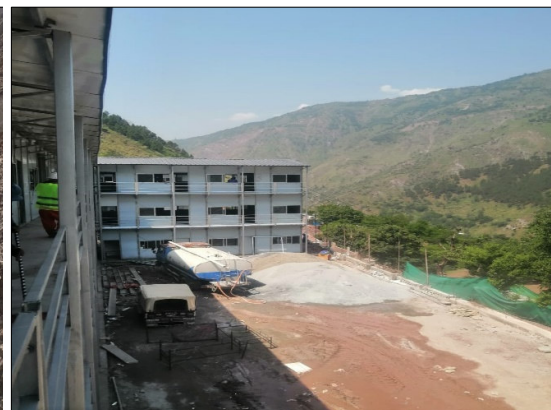
Construction of A3 Camp
