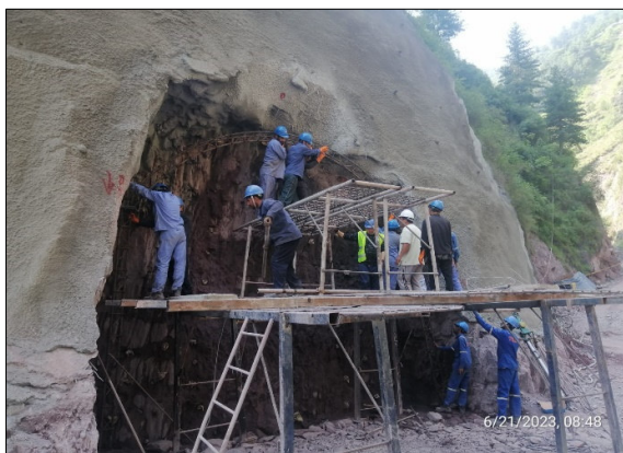
Support work at Adit 2
