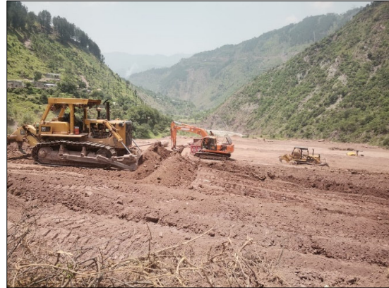
Land leveling at Colony site
