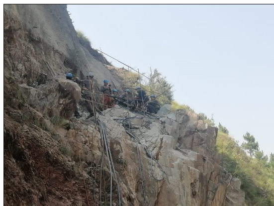
Portal area excavation
