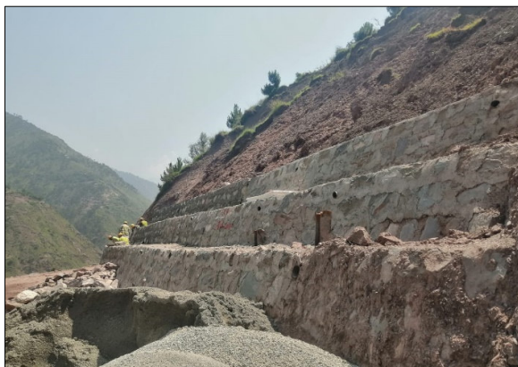
Retaining wall construction at Adit 3
