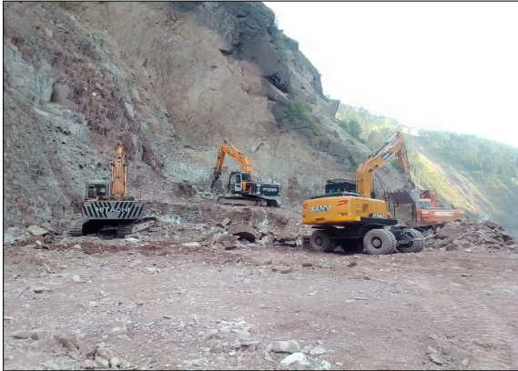
Earthwork at Adit 1
