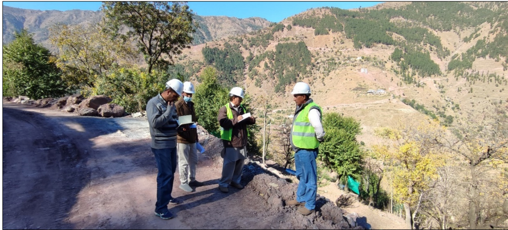
Visit to Temporary Access Road (Adit 3) in connection with the SSEMP review (November 11, 2022)
