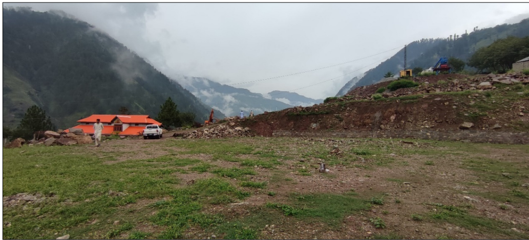
The EPC Contractor's site identified for installation of aggregate plant at Thobi camp site (August 17, 2022)
