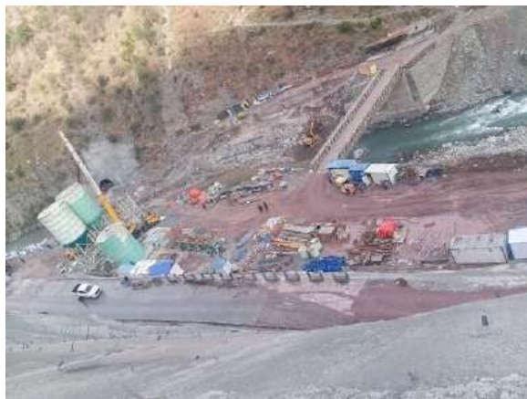
Concrete batching plant installation work at the Dam site
