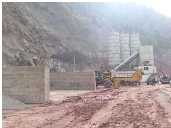
Aggregate storage area of batching plant at the Powerhouse site
