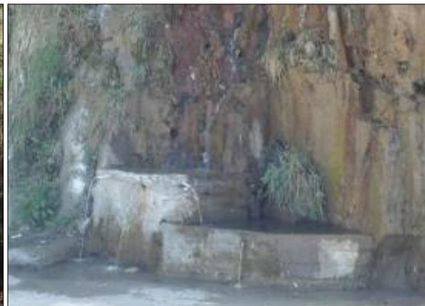
Spring outlet and collection structure at S-10
