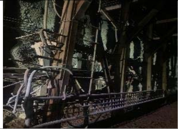
Working platform with improper ladder at main access tunnel
