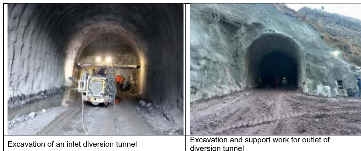
Figure 3-1: Construction of Diversion Tunnel
