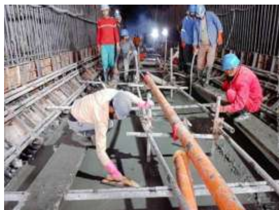
Concrete Pouring in Diversion Tunnel
