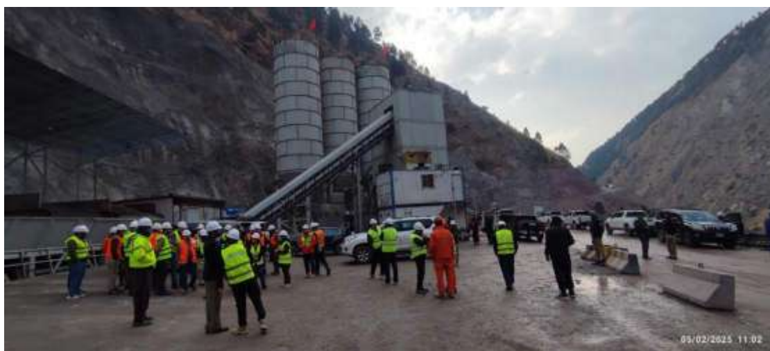
ADB Safeguard Team Visit to the Powerhouse Batching Plant (February 05, 2025)
