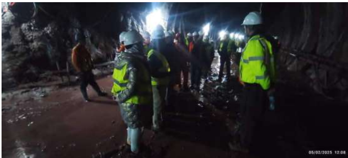
ADB Safeguard team visit to the A3 Adit Tunnel (February 05, 2025)
