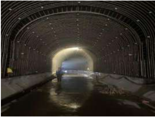
Lining steel in Diversion Tunnel
