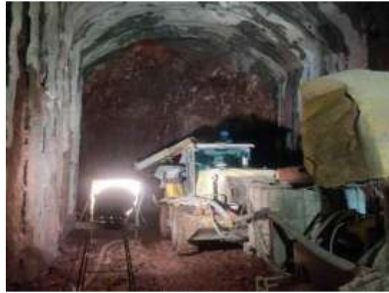
Construction of Main Access tunnel at the Powerhouse site
