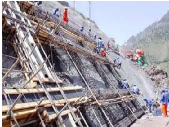
Fixing of Frame beam at the Left Abutment of Dam
