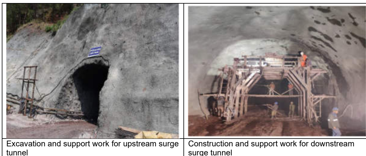
Figure 3-7: Construction work of Surge Shaft, Pressure Tunnel and Power House
