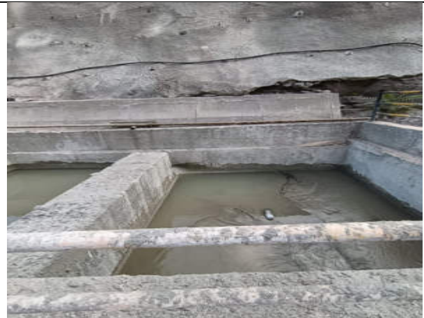
Sedimentation tank of batching plant at dam site is filled with sludge
