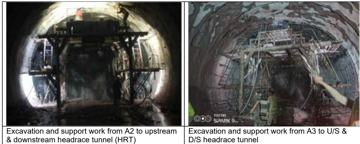
Figure 3-5: Construction of Headrace Tunnel
