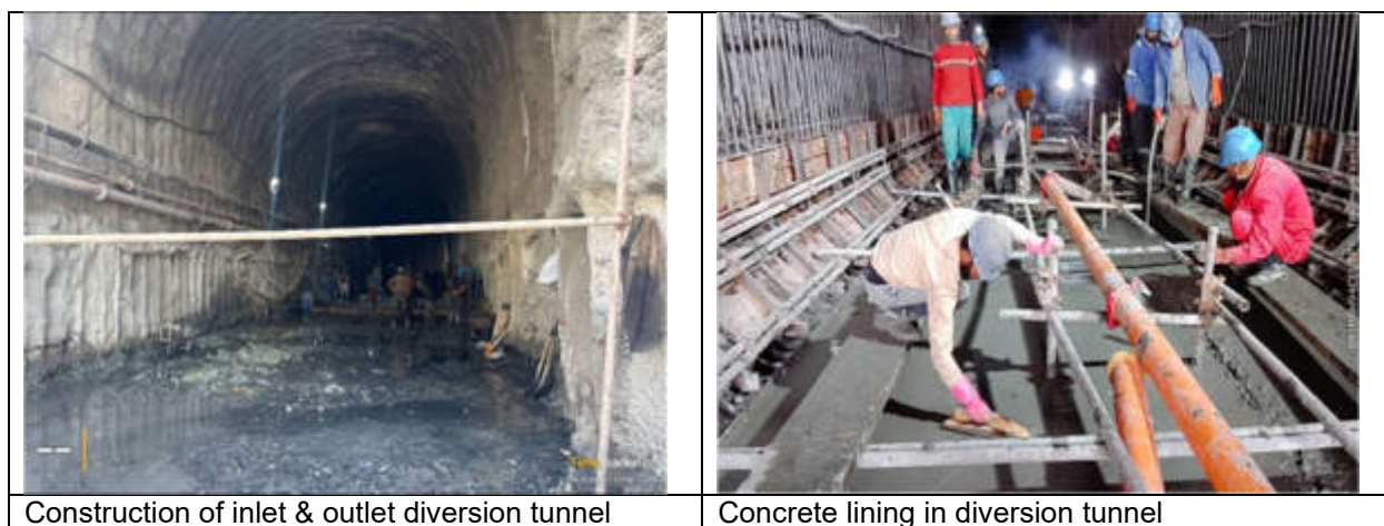
Figure 3-1: Construction of Diversion Tunnel
