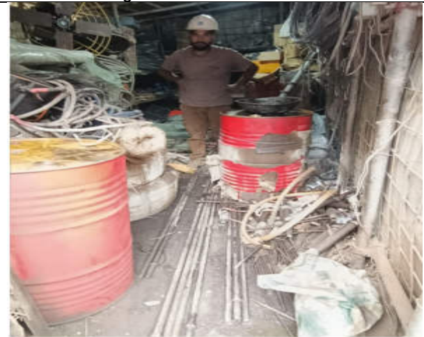
Fuel drum is placed in store- potential risk of fire
