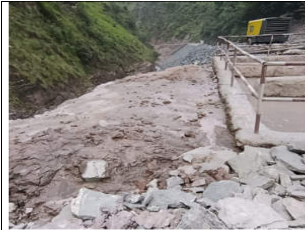
Poor function of sedimentation pond at Adit-2
