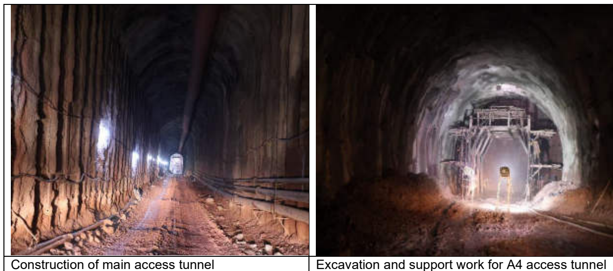
Figure 3-6: Overview of Construction Activities at Main access and Adit Tunnels
