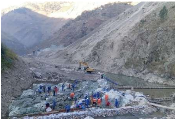
Construction of an upstream (U/S) Concrete Cofferdam
