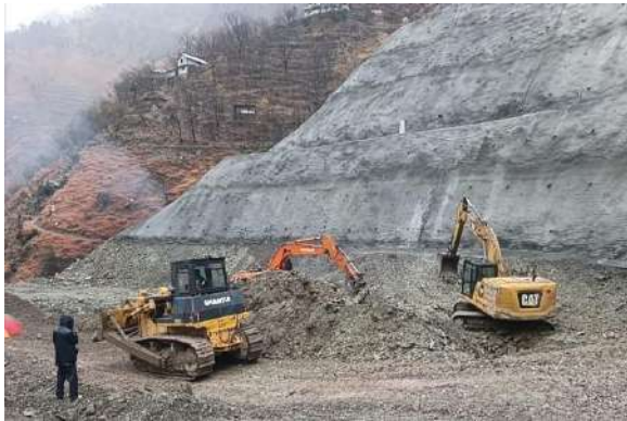
Right Abutment Excavation and Support Works
