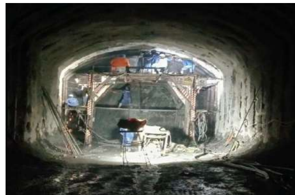
Excavation and Support work at MAT
