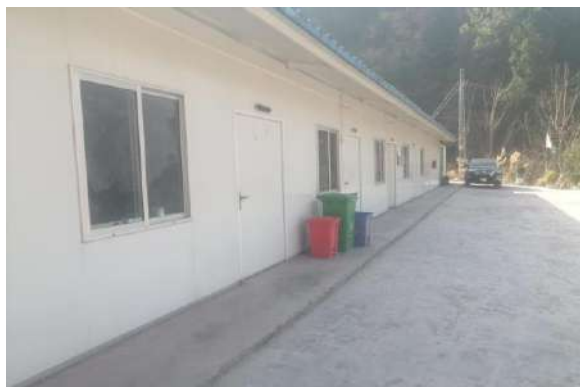
Colored Solid waste bins for the Waste at the EPC GRC Main Camp
