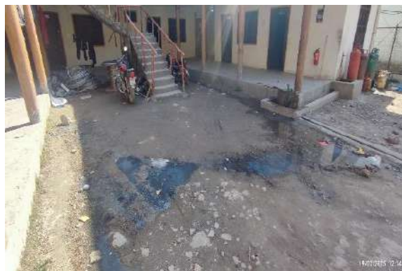
Poor Waste Management in the Pakistani Staff Section of the Main Camp
