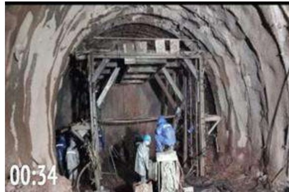
Excavation and Support Works Upstream Surge Tunnel
